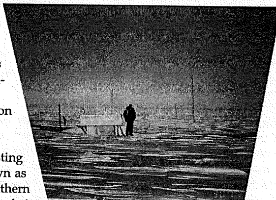
Fig. 36 : Dakshin Gangotri Station as in August, 1990
